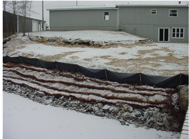
Bank Stabilization Project on the West Branch of the Warroad River
