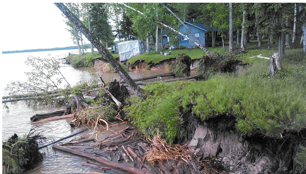
Shoreline erosion on LOW
