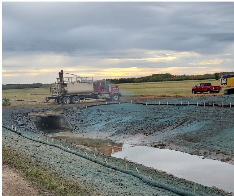
LOW County Ditch One Stabilization Project, Credit: LOW SWCD
