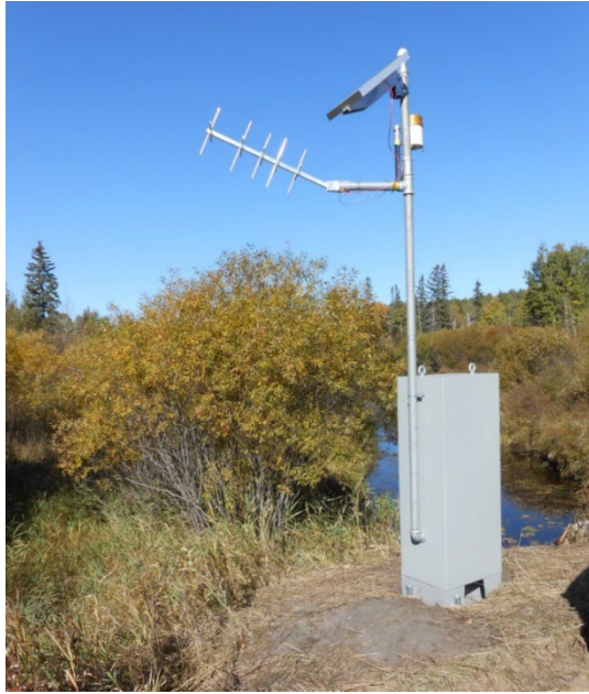
Oaks Monitoring Station
